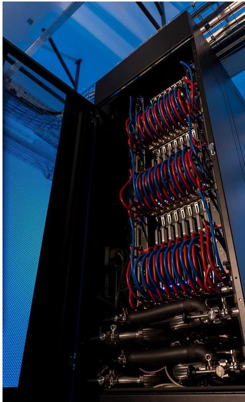
The company MEP designed and implemented a solution that ensures high redundancy and availability of the power and cooling systems for the "Supek" supercomputer, providing a cooling capacity of nearly **100 kW** within a single rack, with very high precision in the inlet temperature of the cooling medium.
